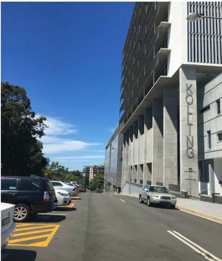
Figure 5: View looking east along Westbourne Street, with Kolling Institute to the south of the site
